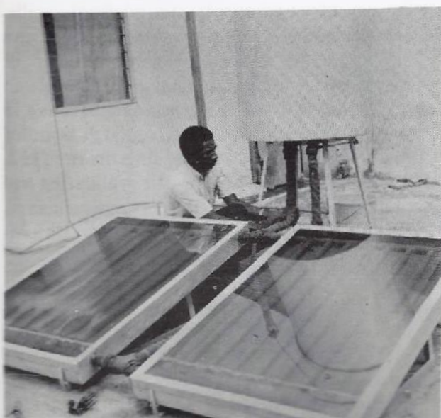
Solar water heater.
