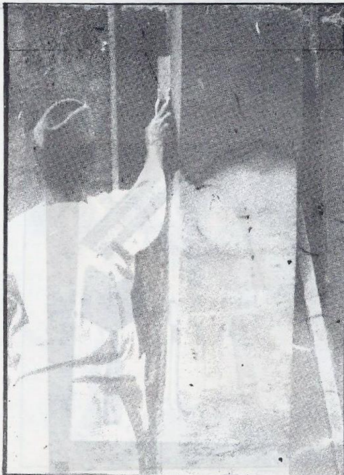
FIG. 15. FINISHING INTERNAL CORNER WITH L-SHAPED GADGET
