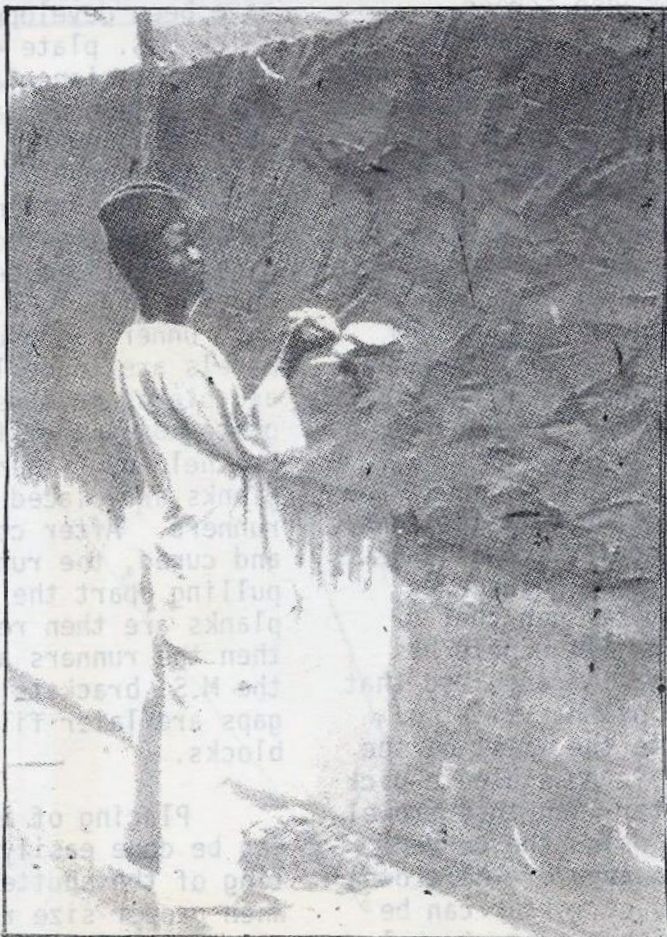
FIG. 11. PLASTERING WITH TRIANGULAR TROWEL
