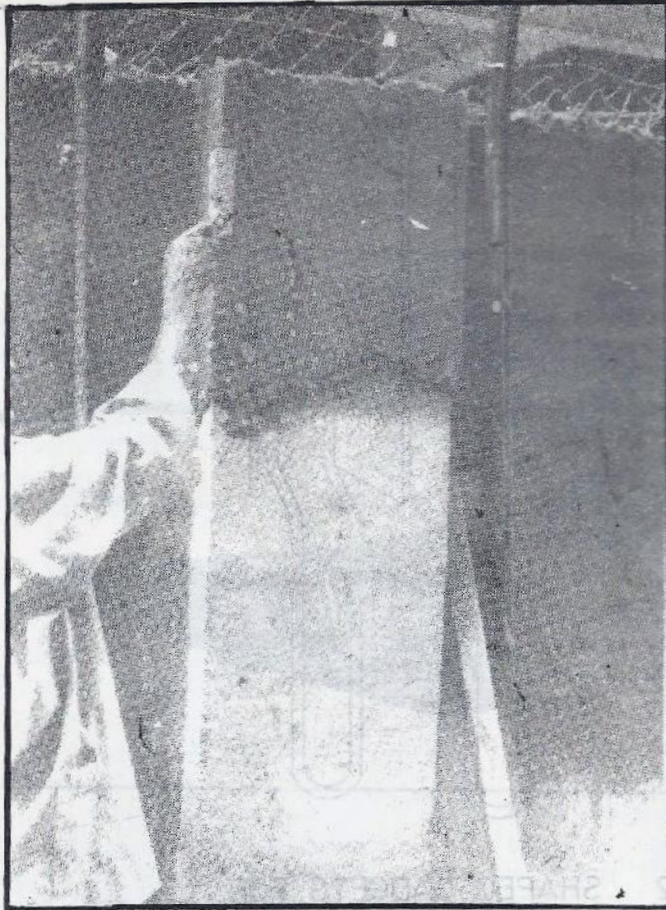
FIG. 14. FINISHING EXTERNAL CORNER WITH L-SHAPED GADGET
