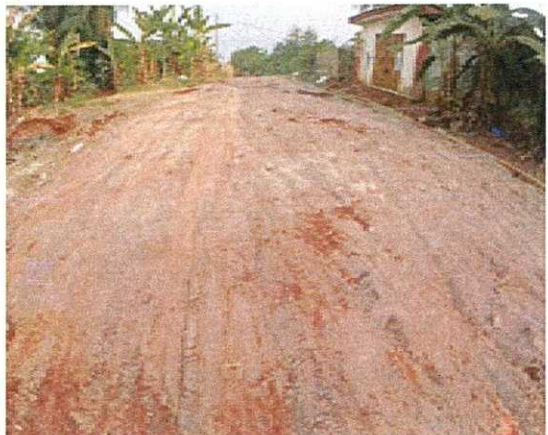
Stabilised erosion prone earth road with modifiers
