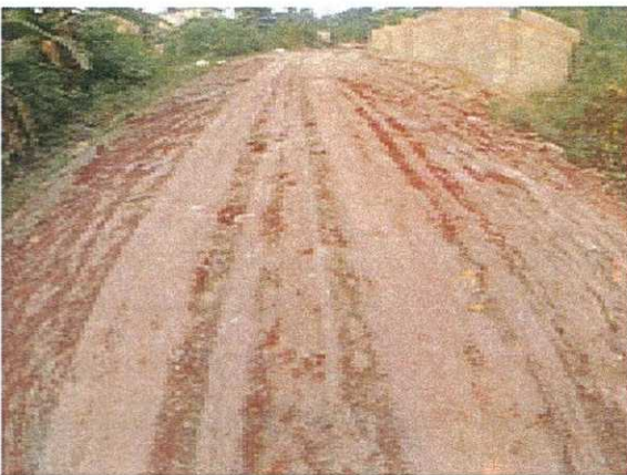
Stabilised erosion prone earth road with modifiers
