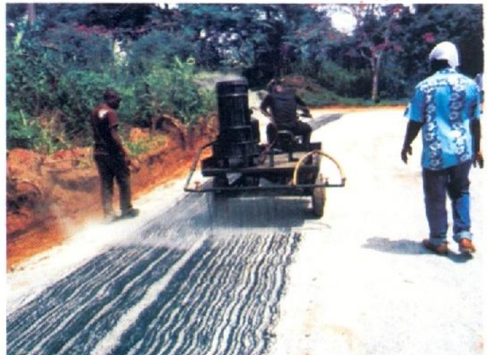
NBRRI Water/bitumen Spraying Machine
