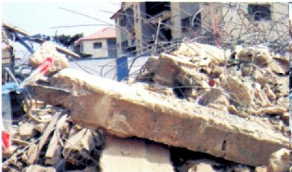
Remnants of Collapsed Building Elements at time of Investigation
