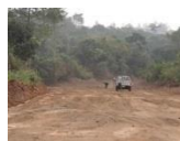
Road construction NLC Ota
