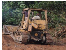
Road construction NLC Ota
