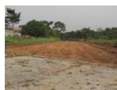
Road construction NLC Ota
