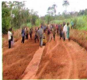
CONSTRUCTION OF RURAL ACCESS ROAD
