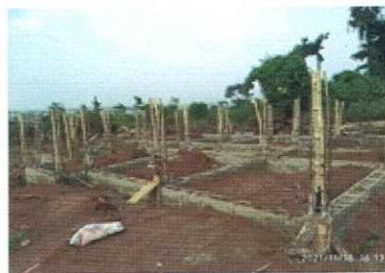
Casting of the Over site concrete floor in progress
