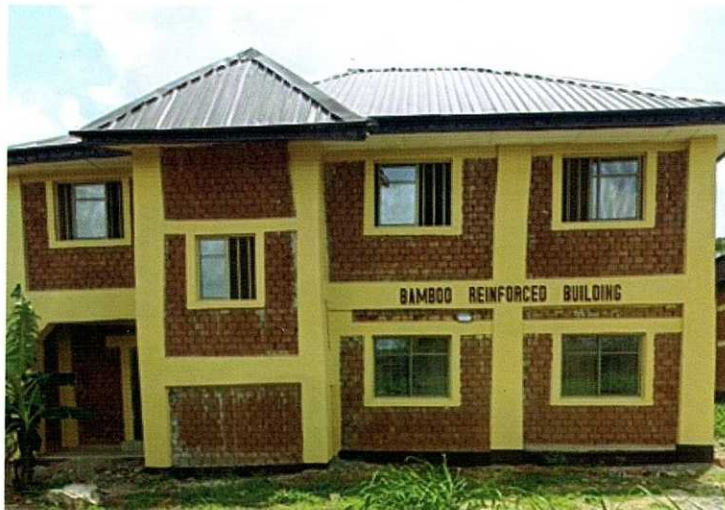
Complete NBRRI storey Building with Bamboo as Reinforcement
