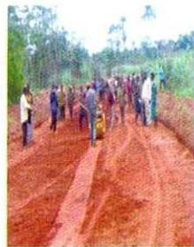
CONSTRUCTION OF RURAL ACCESS ROAD
