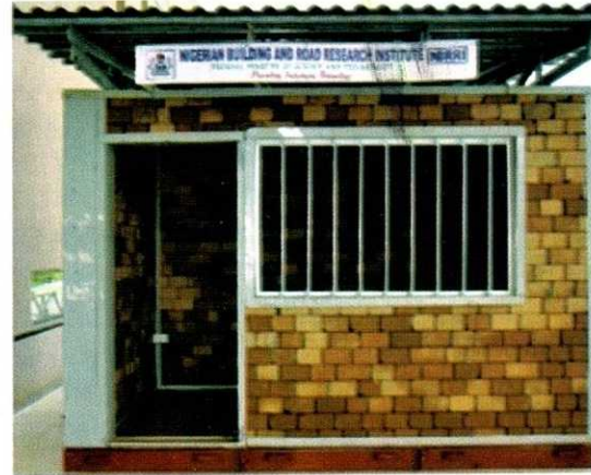
Construction of 1-Room using NBRI'S CSEBs
