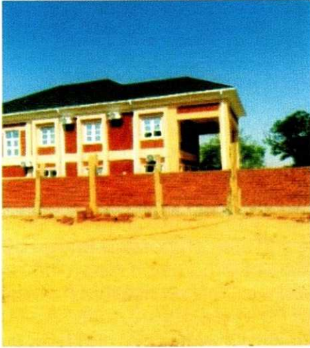
Construction of Duplex using NBRI'S CSEBs
