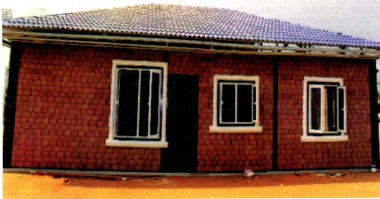
Construction of 3-Bedrooms using NBRI'S CSEBs
