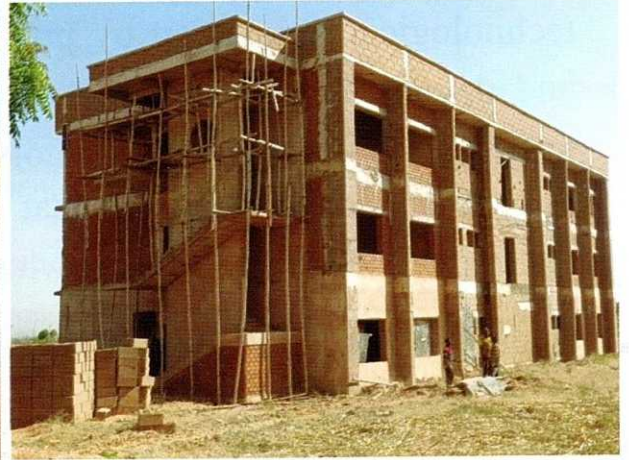
Gombe New Office (Built and own by NBRRI under construction)
