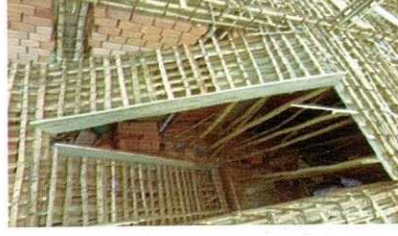
Stair Wall Reinforcement
