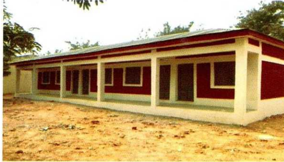
CONSTRUCTION OF BLOCKS OF CLASSROOM IN SELECTED AREAS OF GAYA, AJINGI AND ALBASU FEDERAL CONSTITUENCY, KANO STATE
