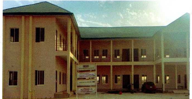
CONSTRUCTION OF AUDITORIUMS, LECTURE HALLS AND OTHER INFRASTRUCTURE IN SOME SELECTED HIGHER INSTITUTION OF LEARNING (COMPLETION OF EDUCATION CENTRE GWAMAI),
