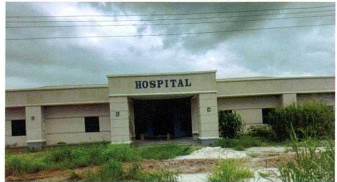
CONSTRUCTION OF WING "A&B" OF STUDENTS HOSPITAL IN FEDERAL POLYTECHNIC, OROGUN, DELTA CENTRAL SENATORIAL DISTRICT, DELTA STATE
