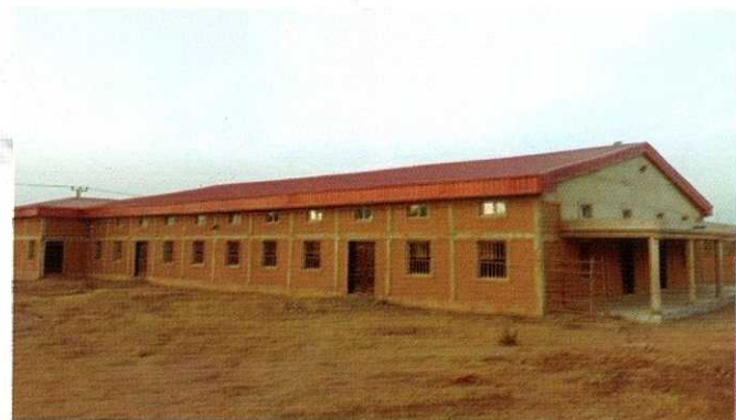
COMMUNITY TOWN HALL TAL, BILLIRI LGA, GOMBE STATE
