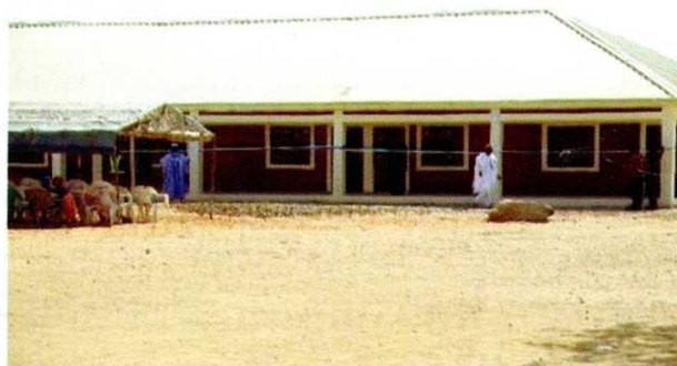
BLOCK OF THREE CLASSROOMS TO THE MANAGEMENT OF ZUL COMMUNITY SECONDARY SCHOOL IN TORO LGA OF BAUCHI STATE
