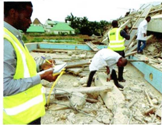
Building Collapse Site (Gwarimpa, Abuja)
