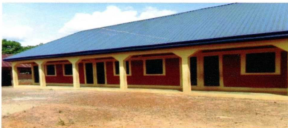
A COMPLETE VIEW OF THE BLOCK OF 3 CLASSROOMS IN COMMUNITY SECONDARY SCHOOL IN IGWELEDOHA COMMUNITY IN IKWO EZZA SOUTH IN EBONYI STATE.
