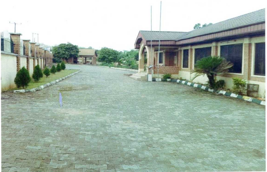
Nnewi Zonal Office undergoing renovation
