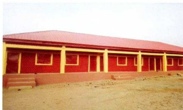
NBRRI COMMISSIONED AND DONATED A BLOCK OF THREE (3) CLASSROOMS AT WAJAH GIRLS PRIMARY SCHOOL IN HONG LOCAL GOVERNMENT AREA OF ADAMAWA STATE.
