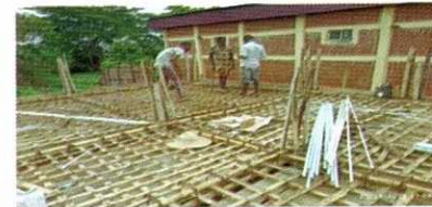
Details of Bamboo Reinforcement on First Floor
