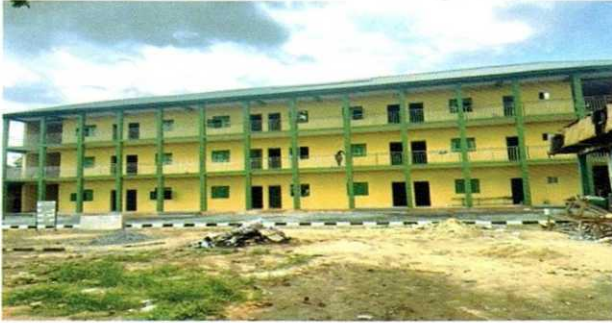
CONSTRUCTION OF CLASSROOMS WITH OFFICE AT 9 BRIGADE PRIMARY SCHOOL, IKEJA
