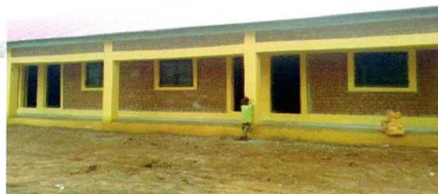
BLOCK OF 3 CLASSROOMS IN GOVERNMENT SECONDARY SCHOOL, GINDIN DOROWA COMMUNITY IN WUKARI LOCAL GOVERNMENT AREA OF TARABA STATE
