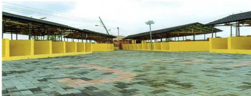
CONSTRUCTION OF MODERN MARKET IN IKORODU FEDERAL CONSTITUENCY,
