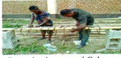
Preparing beams and Columns
