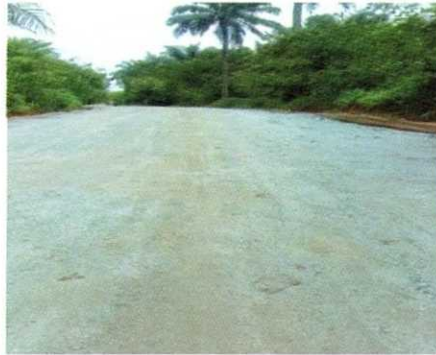
Prepared road surface Natural bituminous (stone base)
