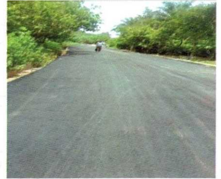
Natural bituminous (stone base) surface at 5, 10 & 15% natural bitumen
