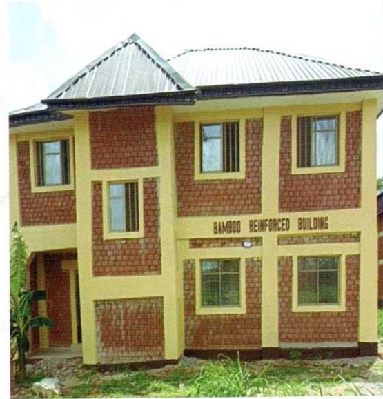
Complete NBRI storey Building with Bamboo as Reinforcement
