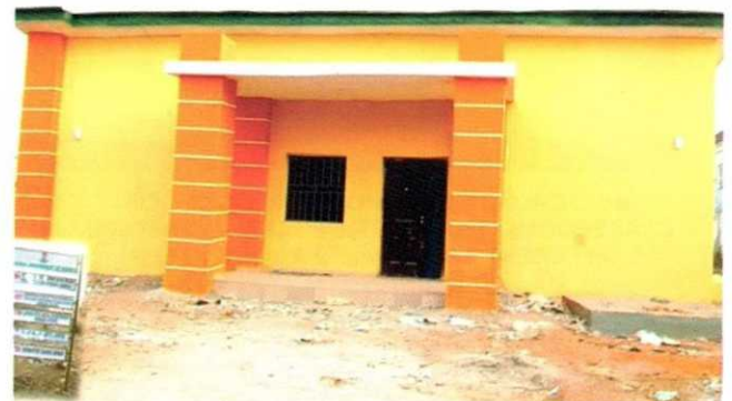
COMPLETION OF FM STATIONS IN EDU AND KAIAMA LGAS.
