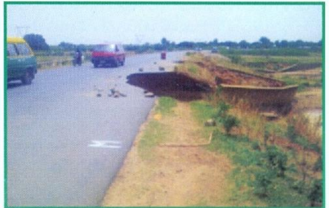
Failed Pavements due to Poor Drainage along some Nigerian roads
