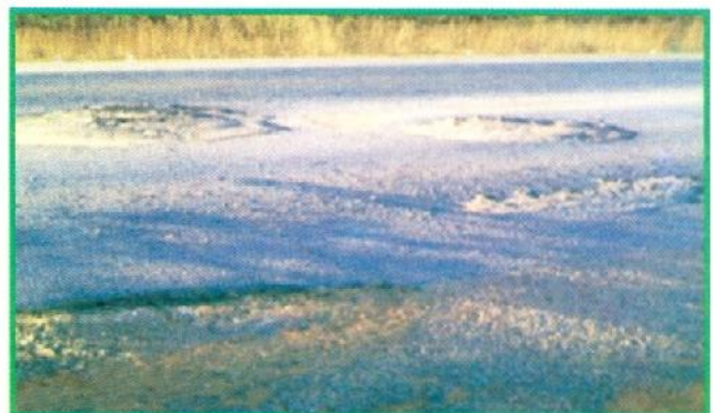
Different types of Potholes on Nigerian roads
