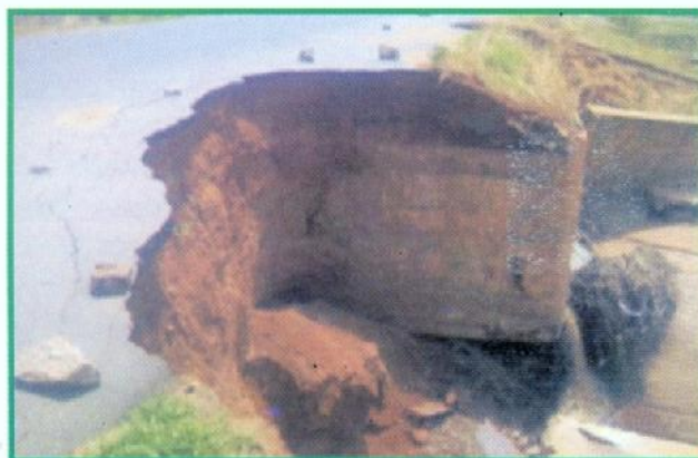
Failed Roadways due to Erosion and Poor Drainage on some Nigerian roads
