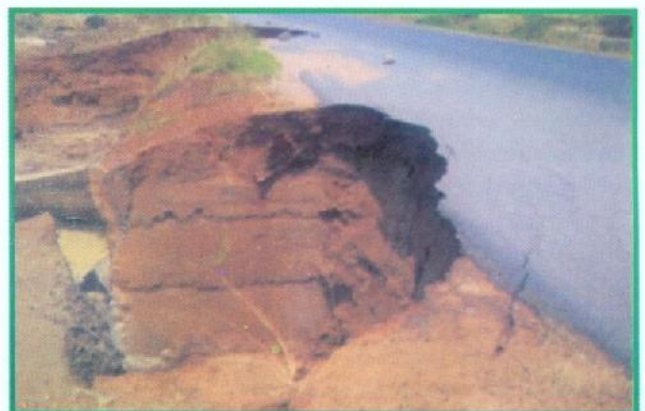
Failed Roadways due to Erosion and Poor Drainage on some Nigerian roads
