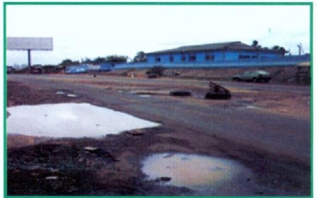
Failed Pavements due to Poor Drainage along some Nigerian roads
