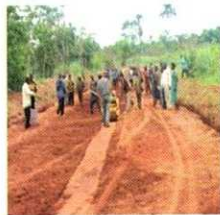
CONSTRUCTION OF RURAL ACCESS ROAD
