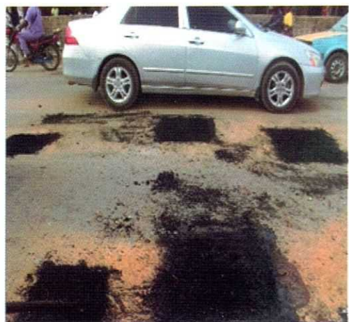
Pothole patching with locally processed bitumen
