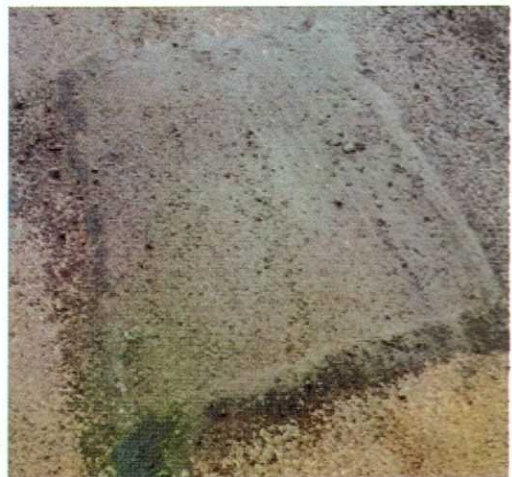
Pothole patching with locally processed bitumen
