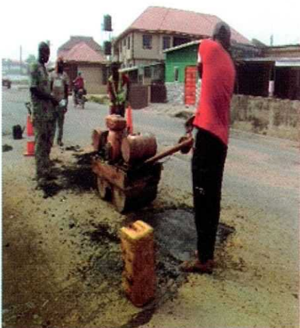
Pothole patching with locally processed bitumen
