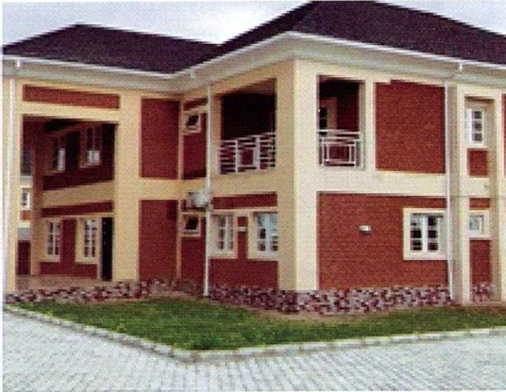
Figure 11: NBRRI Interlocking Brick Application for Duplex Housing in a Nigerian University
