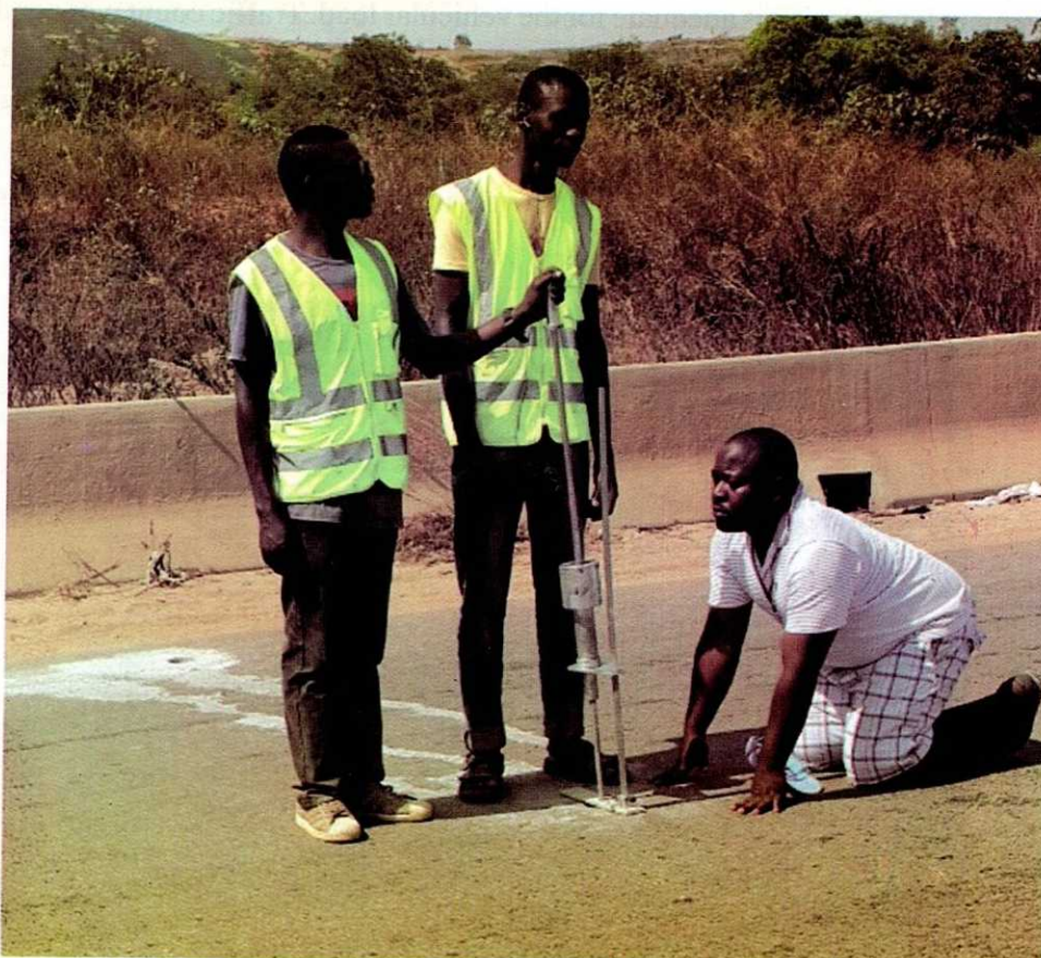
Plate 4: Dynamic Cone Penetration test
