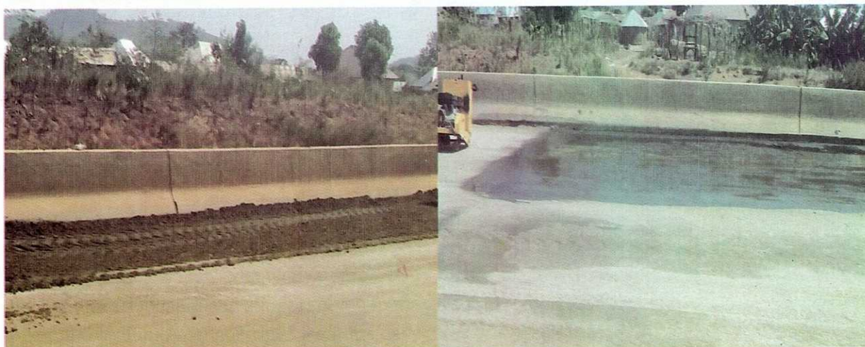
Plate 2: Ongoing rehabilitation works on some sections
