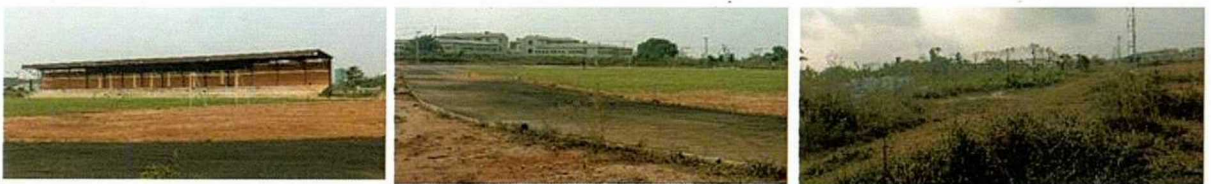
On-going construction of NBRRI Mini Sports Complex in OTA
