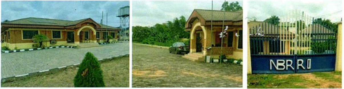
Renovation of the South-East NBRI Zonal Office, Nnewi, Anambra State
