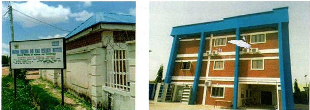
Renovation of the North-West NBRI Zonal Office, Kano
