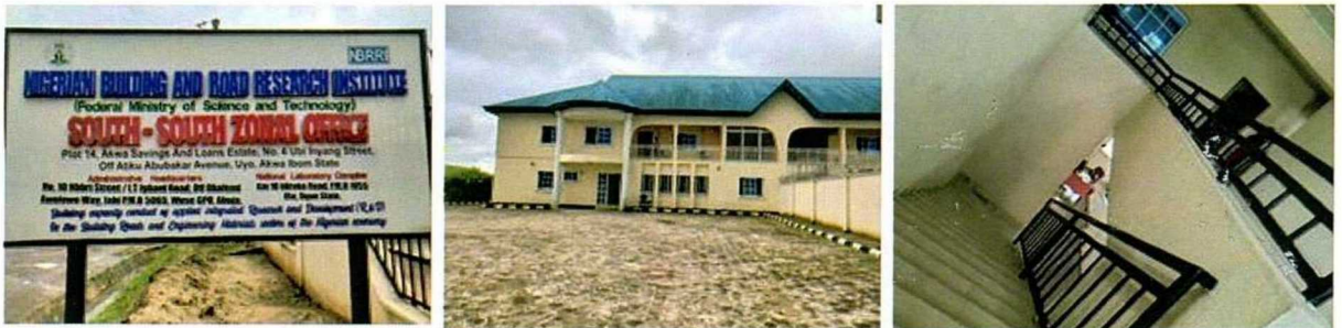
Renovation of the South-South NBRI Zonal Office, Uyo, Akwa-Ibom State
