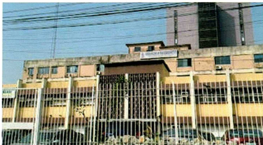
Renovation of the South-West NBRI Zonal Office, Lagos, Lagos State
