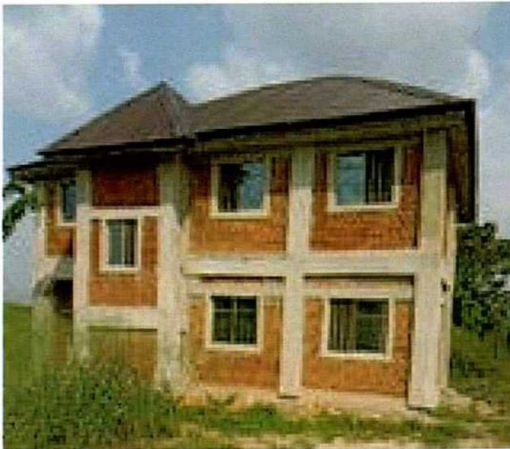
Construction of a Prototype Storey Building with Bamboo as Reinforcements
