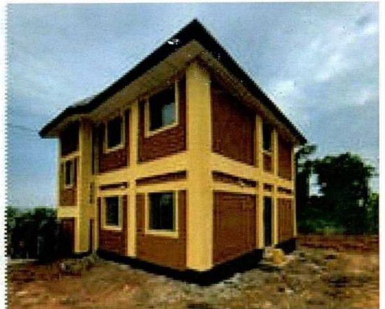
Construction of a Prototype Storey Building with Bamboo as Reinforcements
