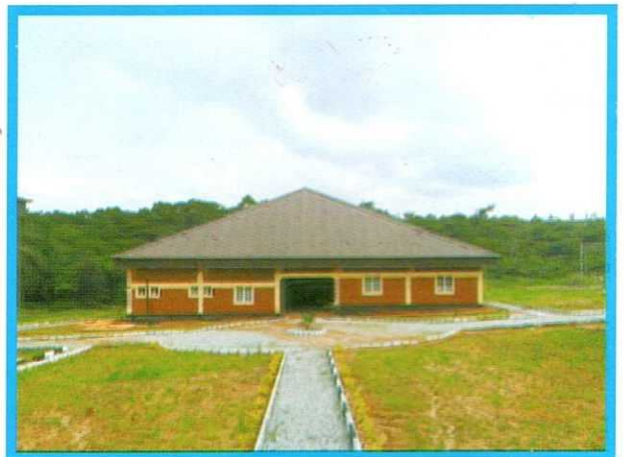
Front view of Block B
