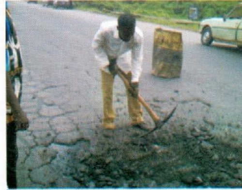
Photo 31 – Using digger to dig out cracked portions of road.
