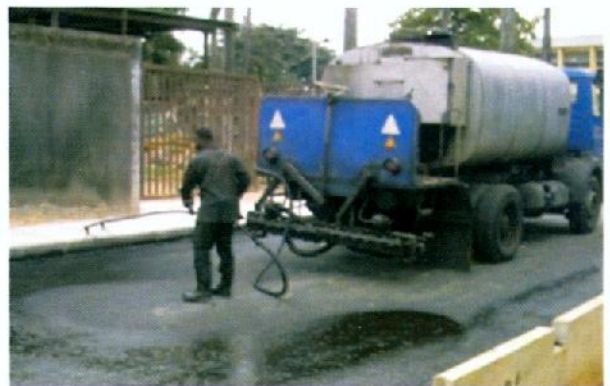
Photo 16 – Spraying tack coat using an extended pressure nozzle
