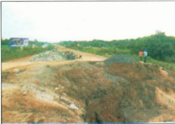
PLATE 9: Reconstruction of collapsed box culvert
