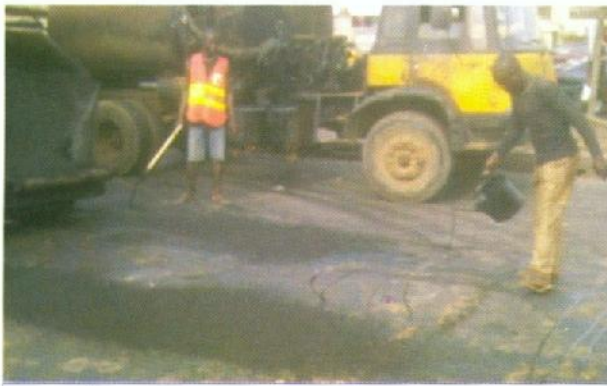
Photo 15 – Applying tack coat to a junction pavement surface using spray can
