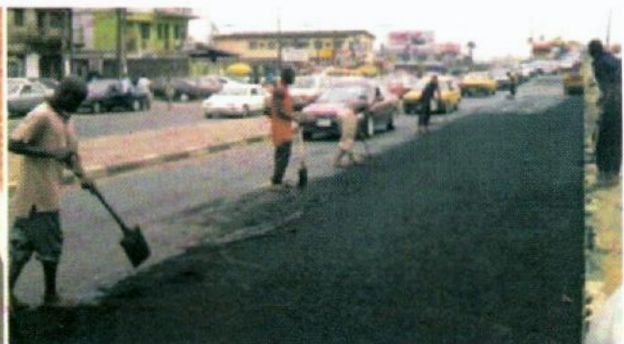
Photo 24 – Using shovels to rake freshly-laid asphalt to level
