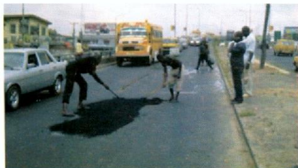
Photo 19 – Filling up localized distressed area with asphalt and raking to level
