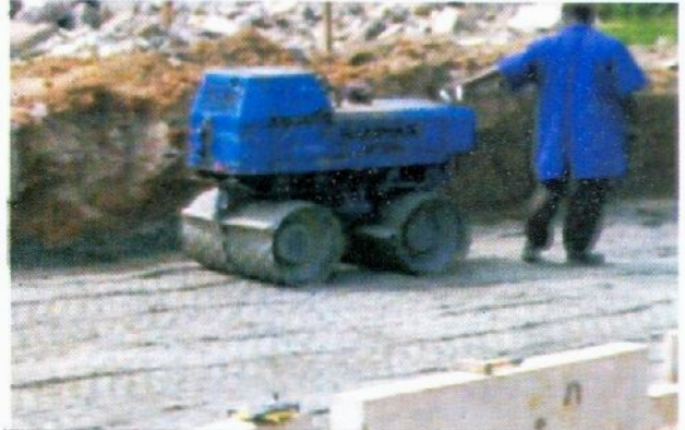
Photo 37 – Compacting stone base using sheep's foot vibratory roller (Courtesy: Julius Berger Nig. Ltd.)
