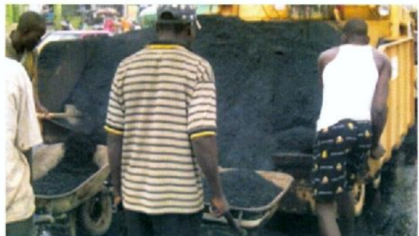
Photo 18 – Taking asphalt from paver to fill localized distressed areas
