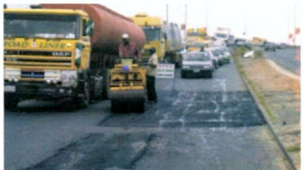
Photo 20 – Compacting patches with vibratory roller
