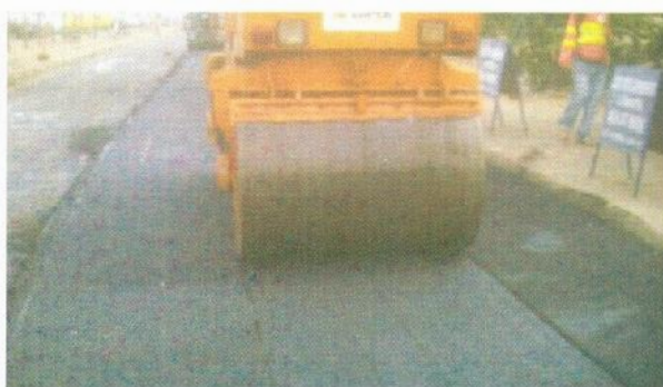
Photo 26 – Compacting freshly-laid asphalt using vibratory steel drum roller
