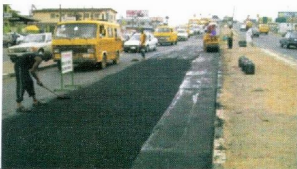
Photo 25 – Commencement of compaction of freshly-laid asphalt concrete
