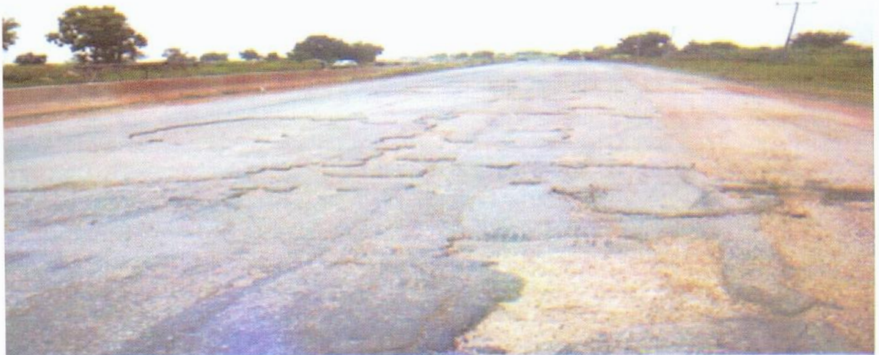
Figure 7: Delamination
