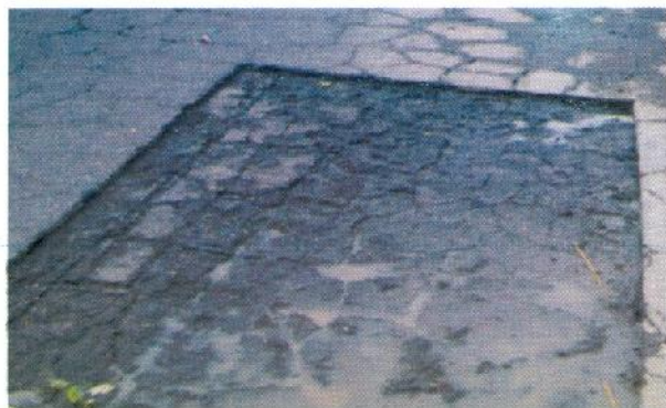
Photo 32 – Close-up view of scarified pavement down to binder course level only.
