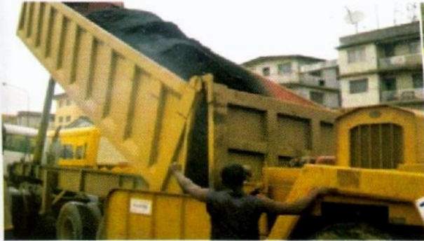
Photo 21 – Tipping stockpiled asphalt into the paver bucket
