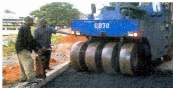
Photo 27 – Finish-compaction of freshly-laid asphalt using pneumatic-tyre roller
