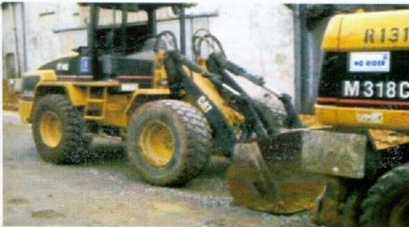
Photo 38 – A typical bulldozer used to scarify road pavement
