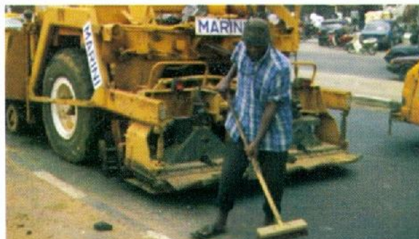
Photo 8 – Cleaning surface of pavement with long broom before overlay activities
