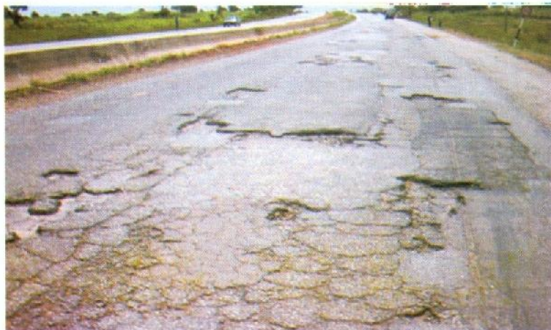
Figure 6: Slippage cracks
