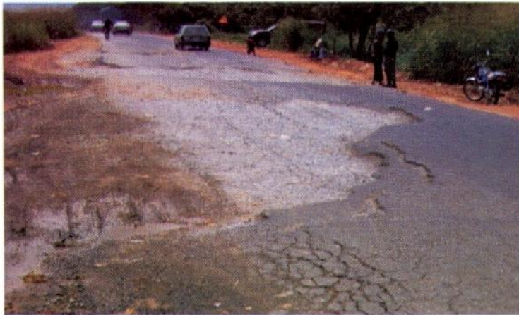
Figure 5: Edge Cracking
