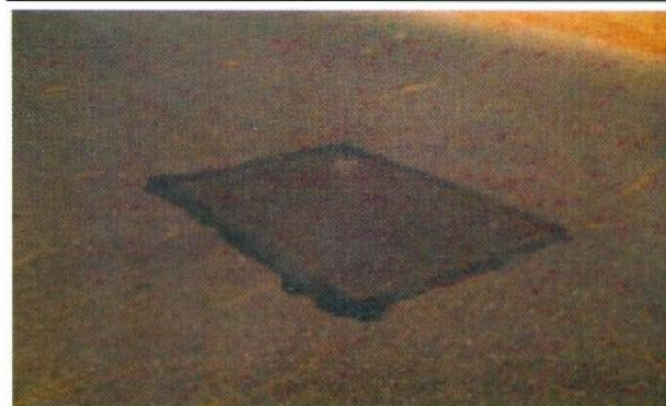
Photo 35 – Close-up view of rehabilitated road section.
