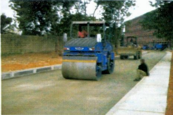
Photo 36 – Compacting stone base with vibratory roller (Courtesy: Julius Berger Nig. Ltd.)
