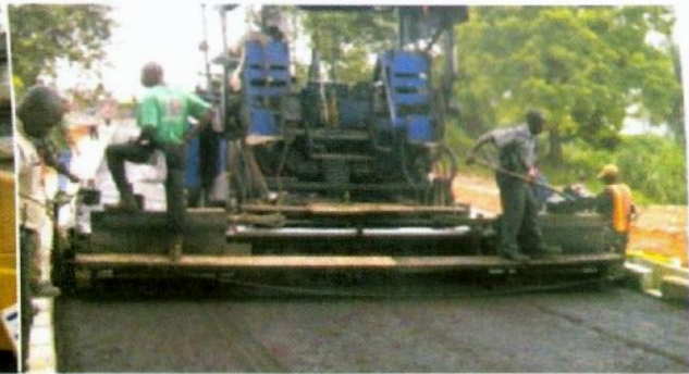
Photo 22 – An asphalt paver laying fresh asphalt wearing course
