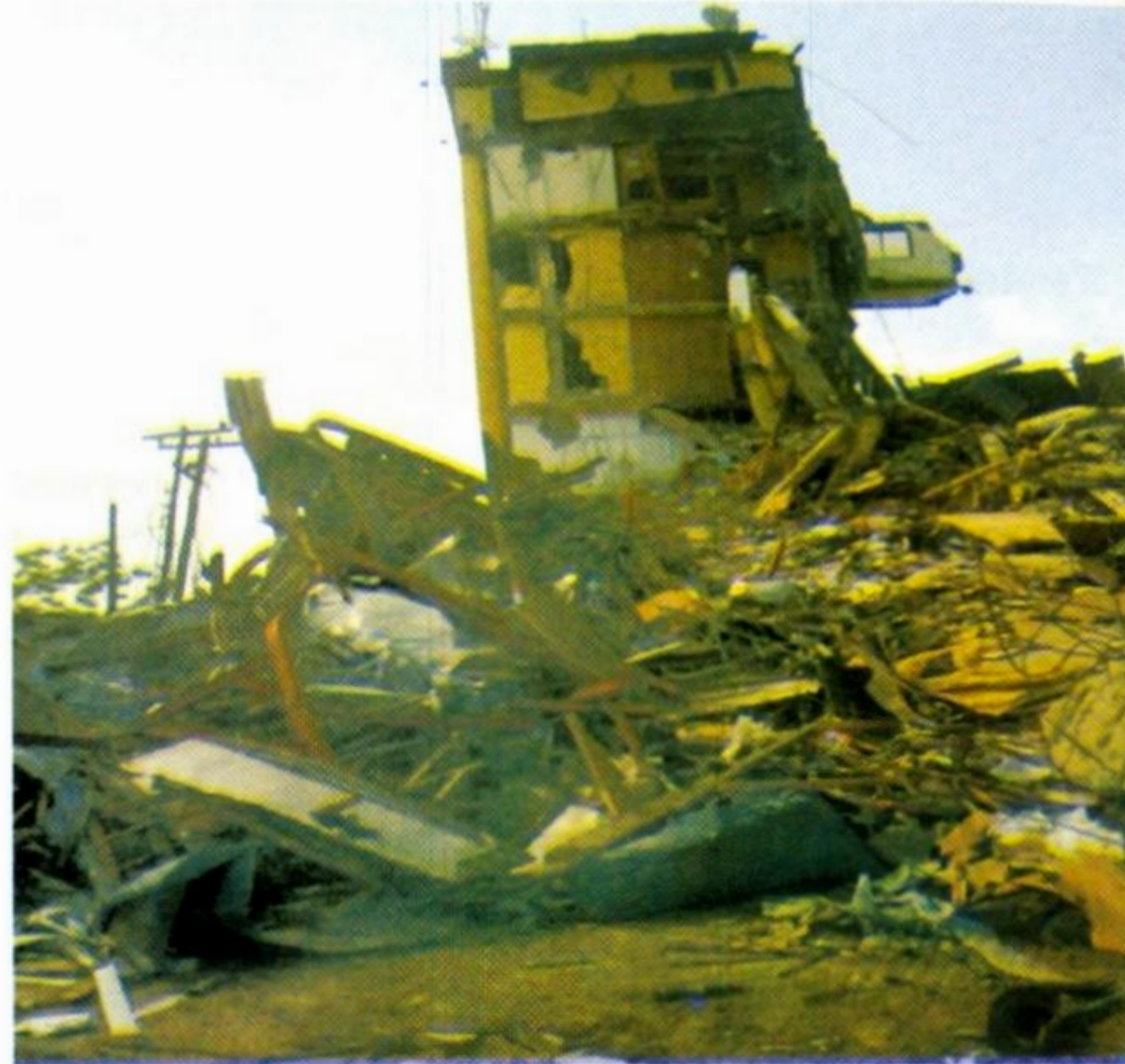
Figure 2: Collapse of 6-Storey Building at MaryLand, Lagos, 26 th October 2011
