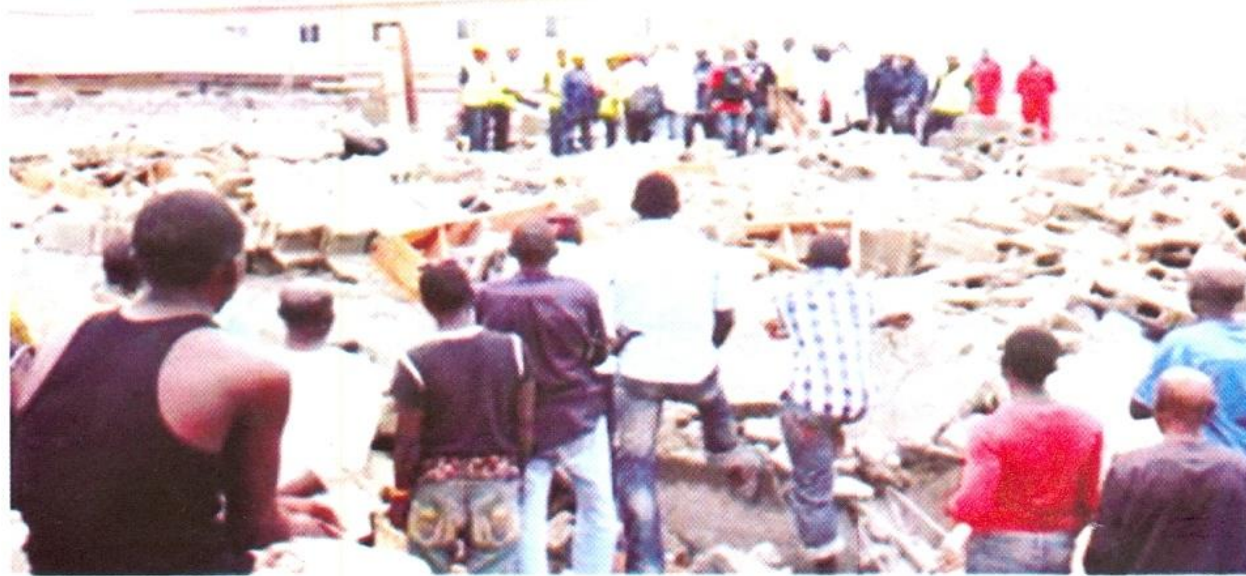
PLATE 7: COLLAPSE OF A TWO STOREY BUILDING OWNED BY NIGERIAN NAVY IN GWARIMPA, ABUJA
