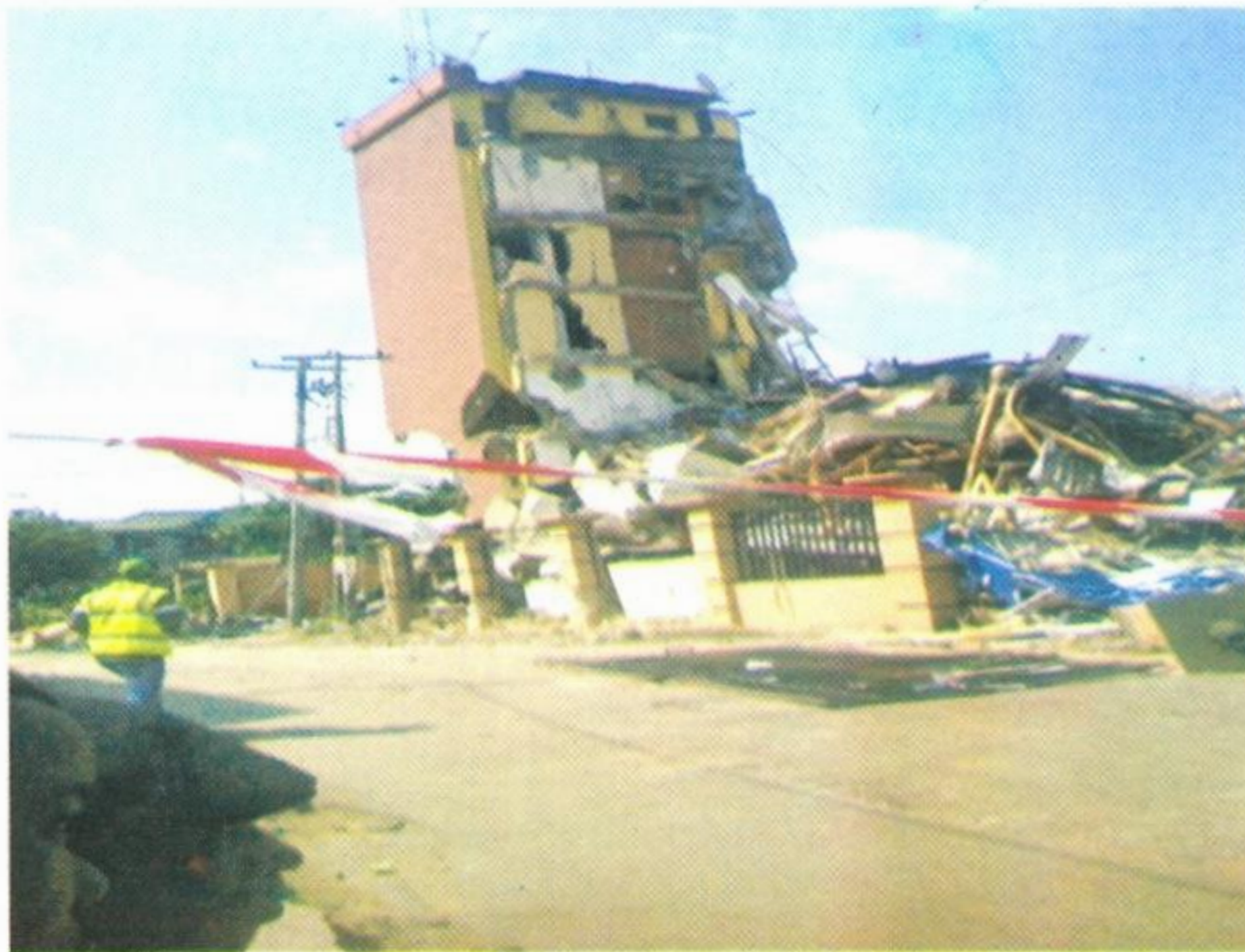
PLATE 4: COLLAPSED 6 (SIX) STOREY BUILDING IN LAGOS
