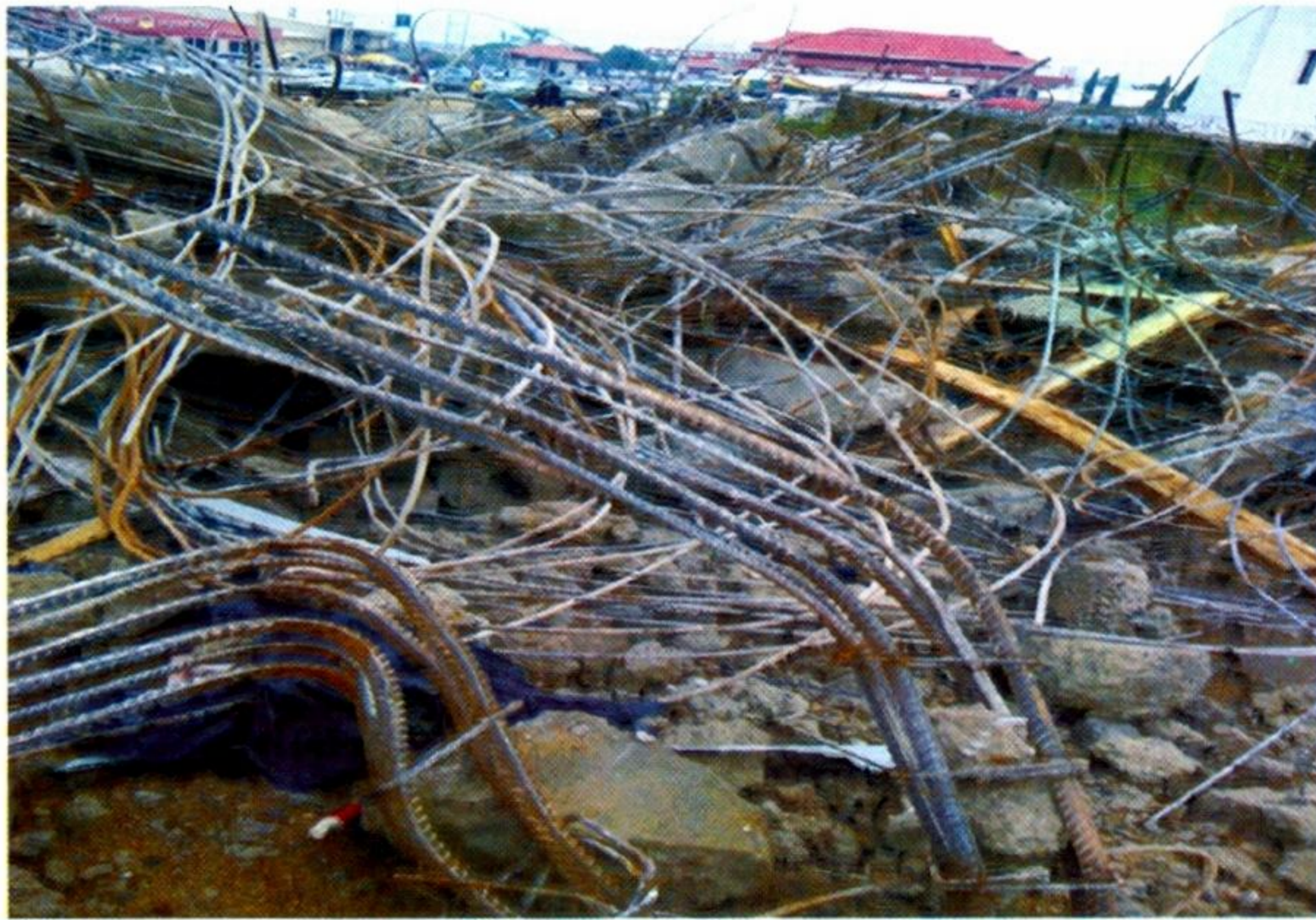
Figure 3: Two Storey Zenith Bank Collapse at Mararaba, Abuja outskirts, 5 th July 2011
