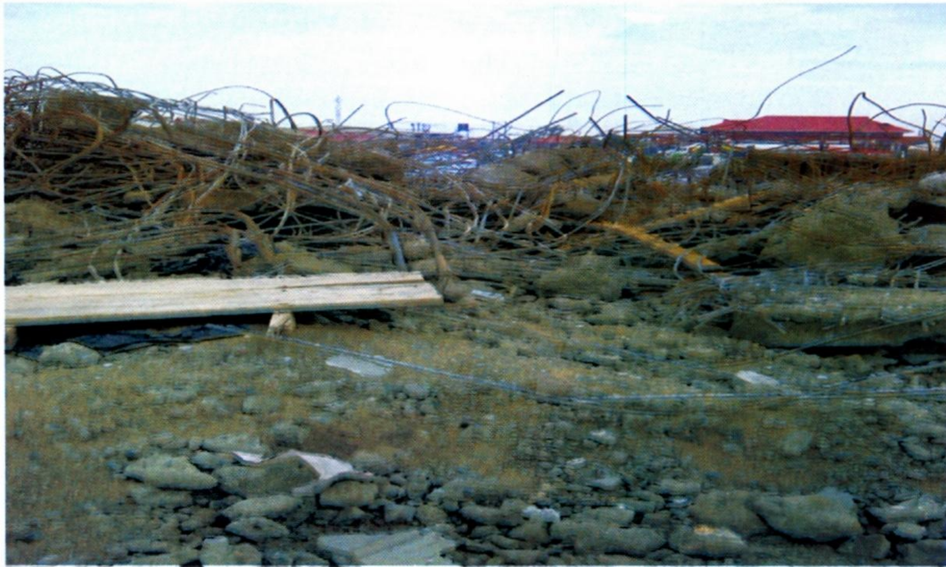
Figure 4: Disintegrated Building, Mararaba, Abuja outskirts, 5th July 2011
