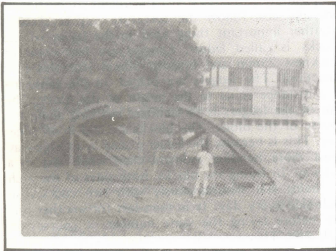
PLATE III – LAYING CLOSE TO CROWN
