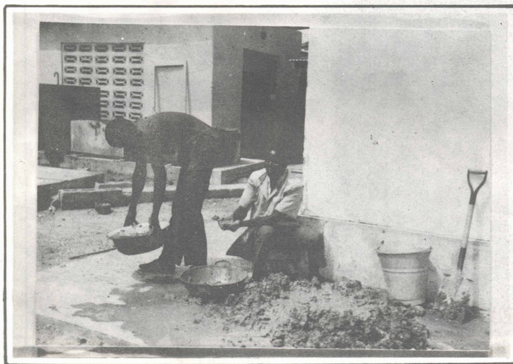
Fig. 8: Preparation of Mud Mortar
