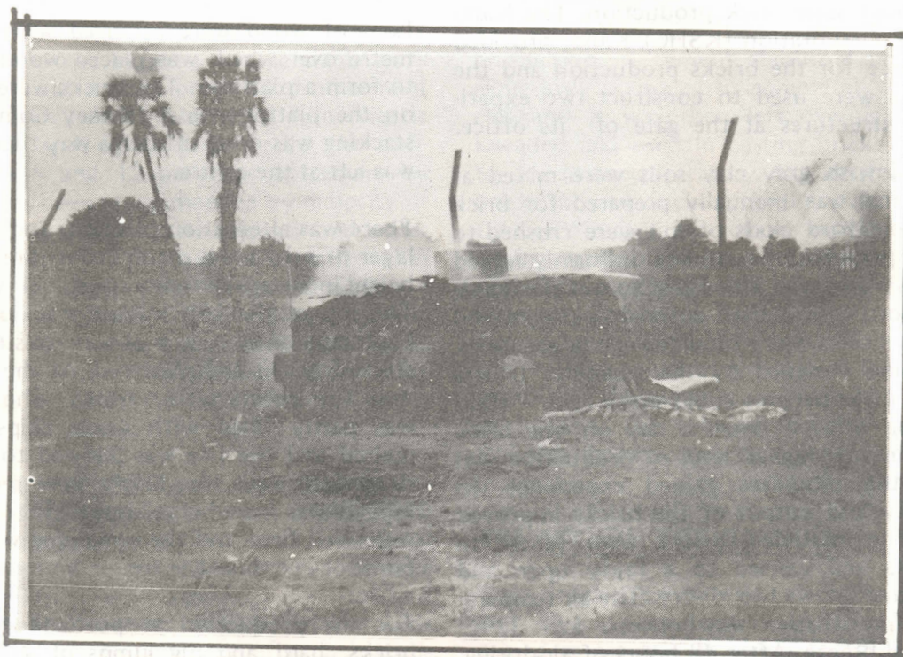
Fig. 5: Firing Bricks in a Clamp Kiln.
