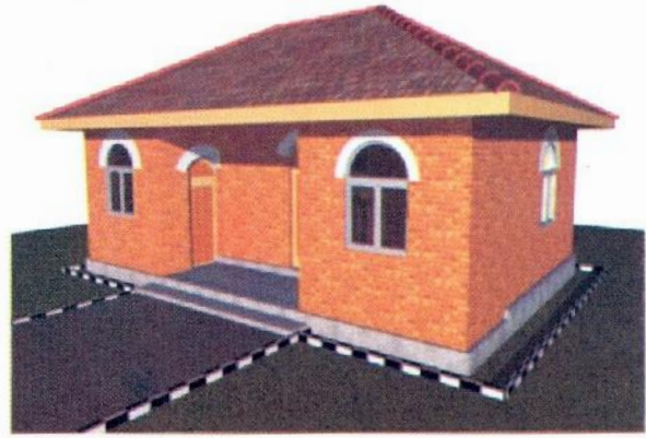
Figure 15: Building with rendered corbel arches replacing lintels.
