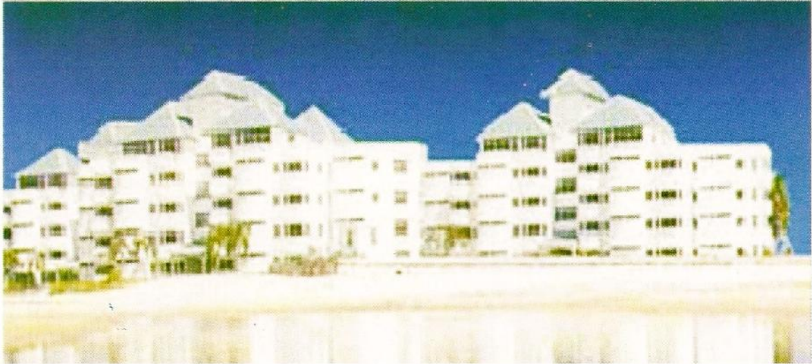
Figure 1 : View of Condominiums in Malaysia
